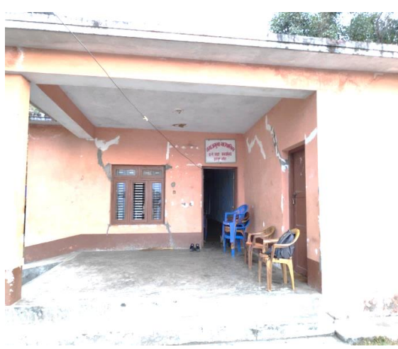
Office Building of Ward 7
