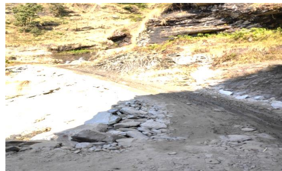
A typical road section from the RM
